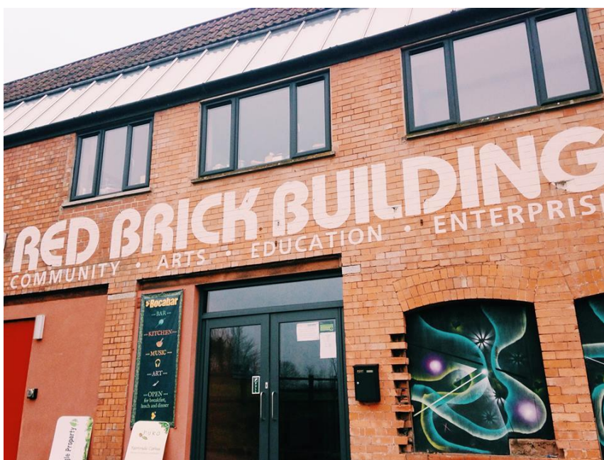
Buildings A and B
